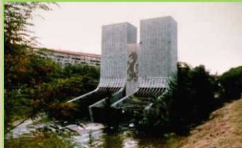
Portal of the Fourvière Tunnel – Lyon ( France)
