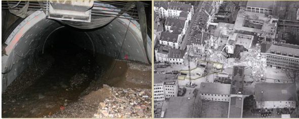
Courtesy WDR Running tunnel filled with inflow material
