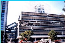
Severe damage to the City Hall
