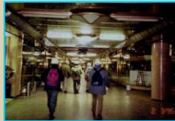
Almost no damage to the underground shopping mall
