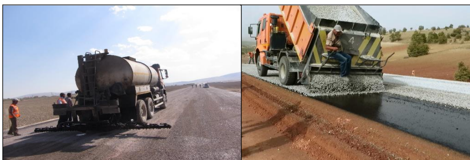
Figure-2: Primer Binder and Surface Coating Application
