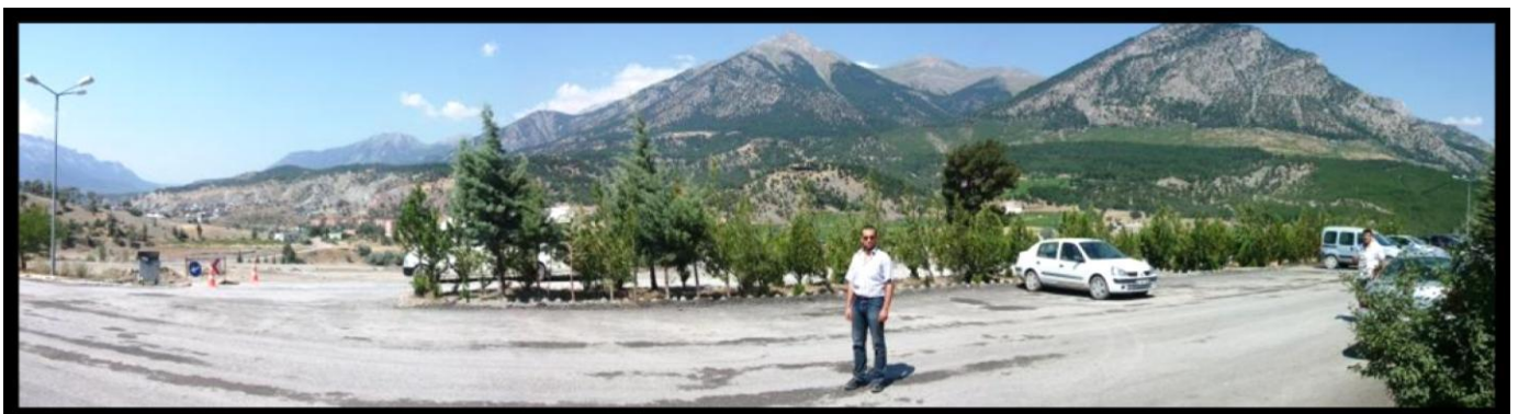
Panoramic view of Pozanti construction site
