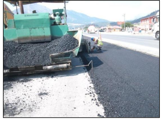
Pozanti road construction
