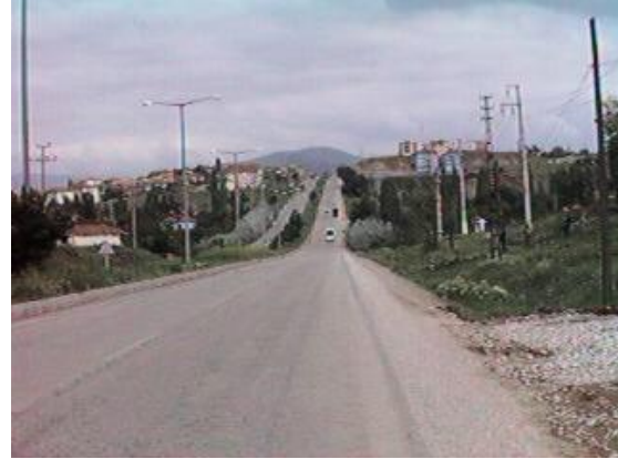
Road 765 through Kırşehir, south part
